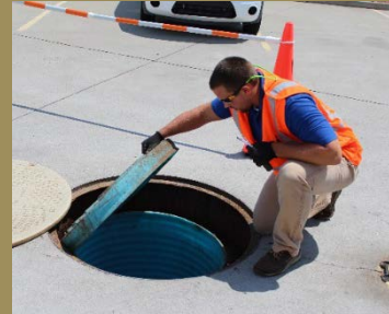
Inspecting a containment sump
