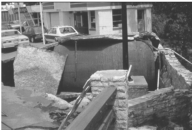
UST lifted by buoyant force
