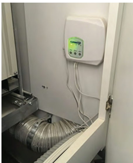
A water leak detection system like this one will alarm if the water level gets too high.
